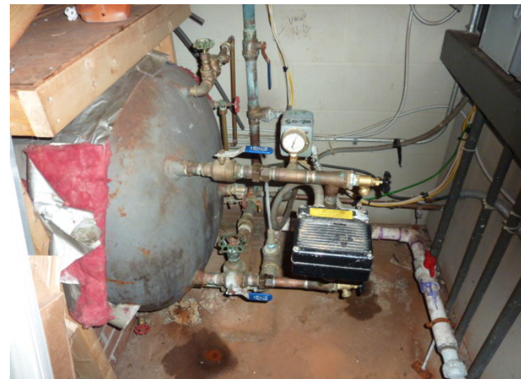
Domestic water storage tank in the Community Building is served by adjacent on-site well.
