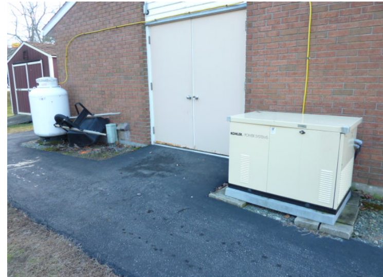
Gas-fired emergency generator and tank at the Community Center.
