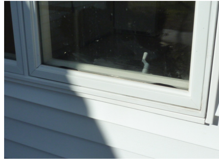
Typical gasket failure at original windows.
