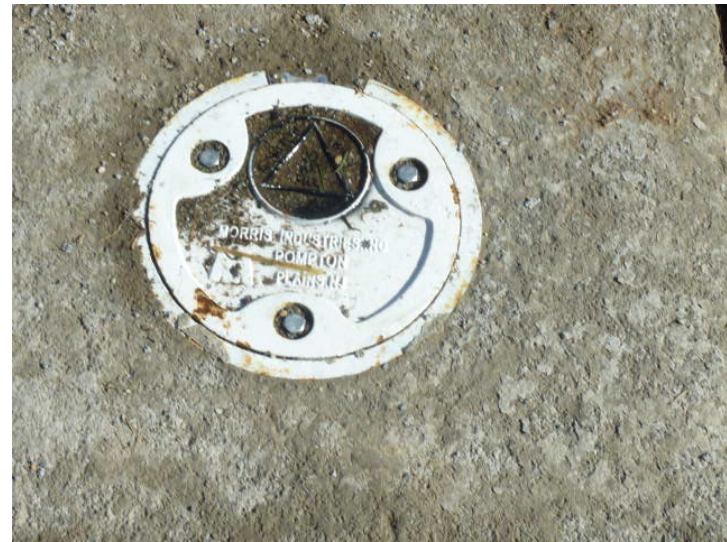
One of 5 monitoring wells installed by the State of CT to evaluate ground water down gradient from the gas station on the adjacent site to the east.
