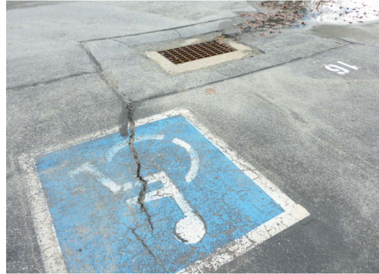
Typical asphalt drives failure.
