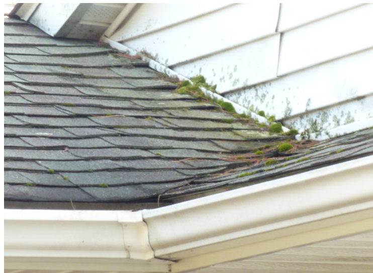
Organic growth on asphalt shingle roofs at select locations.
