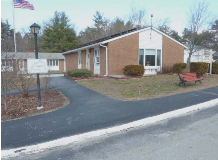
Asphalt walks at the Community Center are generally in good condition; asphalt paving elsewhere at drives, walks and curbs are generally in poor condition.
