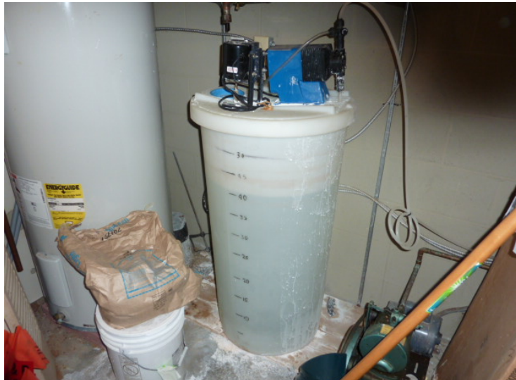
Tank for maintenance of proper PH level in domestic water from on-site well.
