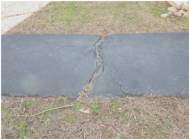
Typical asphalt walks failure.
